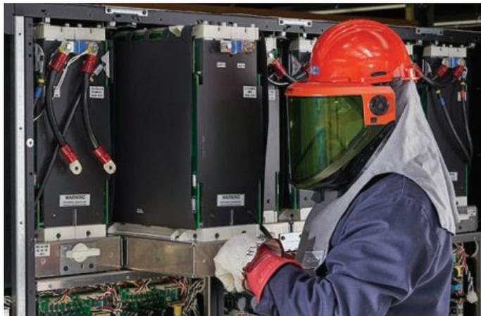
The Power Xpert 9395 is easy to service with 100 percent of the components accessible from the front and an inverter section that only requires releasing two cables and twisting the lever to release.
